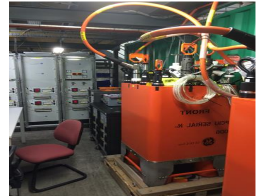
Test Setup Subsea
